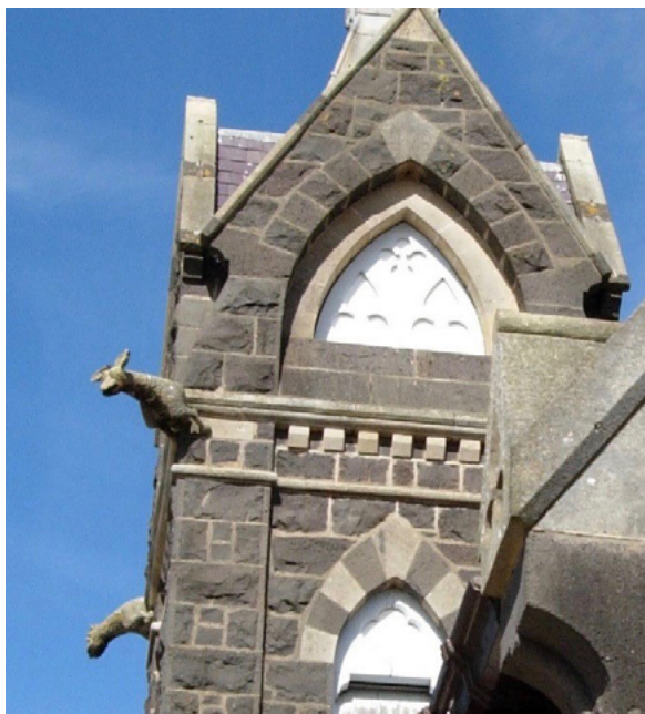
Figure 11: Gargoyles at St Andrew's Presbyterian Church, Skipton, architects Davidson and Henderson, erected 1871. Photographer Allan Willingham (Courtesy Allan Willingham, 'Two Scots in Victoria: The Architecture of Davidson and Henderson', M.Arch. thesis, University of Melbourne, 1983, p. 287)
