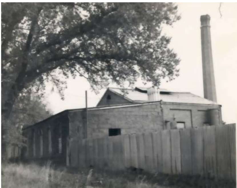
Figure 1: The Praagst gasworks in Kyneton, unchanged in form after being converted to use coal in place of gum leaves (Courtesy National Trust of Australia (Victoria) Database, B1272)
