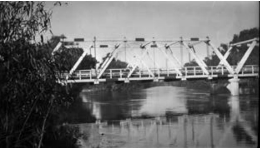
Figure 2: The Union Bridge over the Murray River connecting Wodonga in Victoria and Albury in NSW in 1918 (Courtesy Victorian Public Record Office, VPRS17684/P0003/976, 18_00059)
