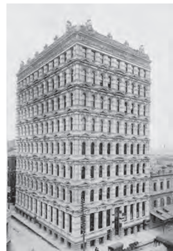
Prell's Building, south-east corner of Queen Street and Flinders Lane, c. 1890 RHSV A-470.002
