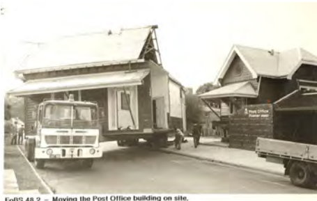
FoBS 48.2 – Moving the Post Office building on site.
