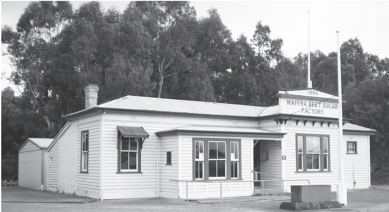
Former Sugar Beet Factory occupied by the Maffra Historical Society. Image courtesy of the Maffra and District Historical Society.
